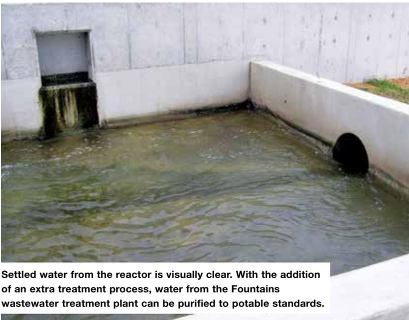
**Settled water from the reactor is visually clear. With the addition of an extra treatment process, water from the Fountains wastewater treatment plant can be purified to potable standards.**
