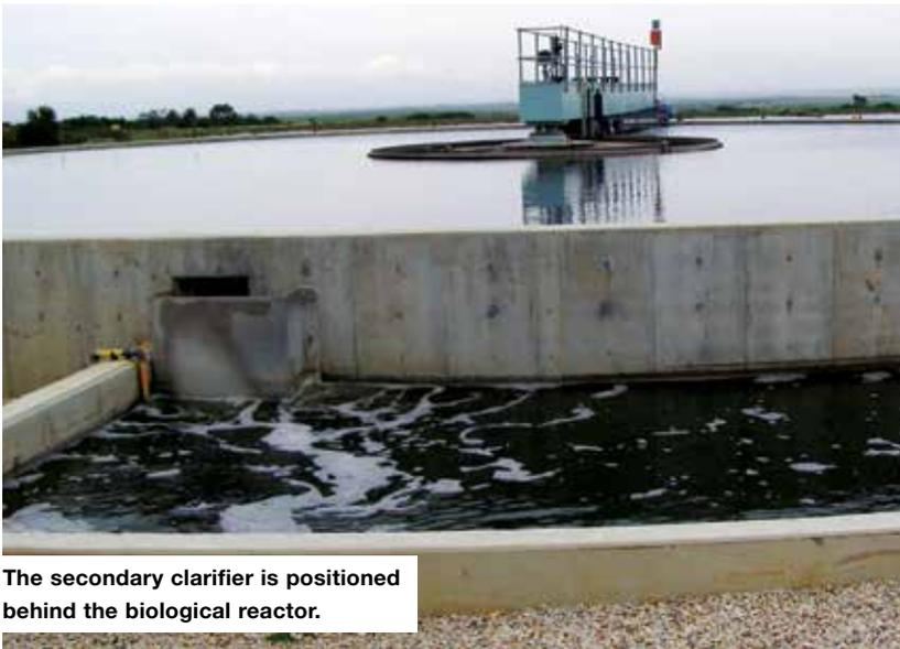
**The secondary clarifier is positioned behind the biological reactor.**
